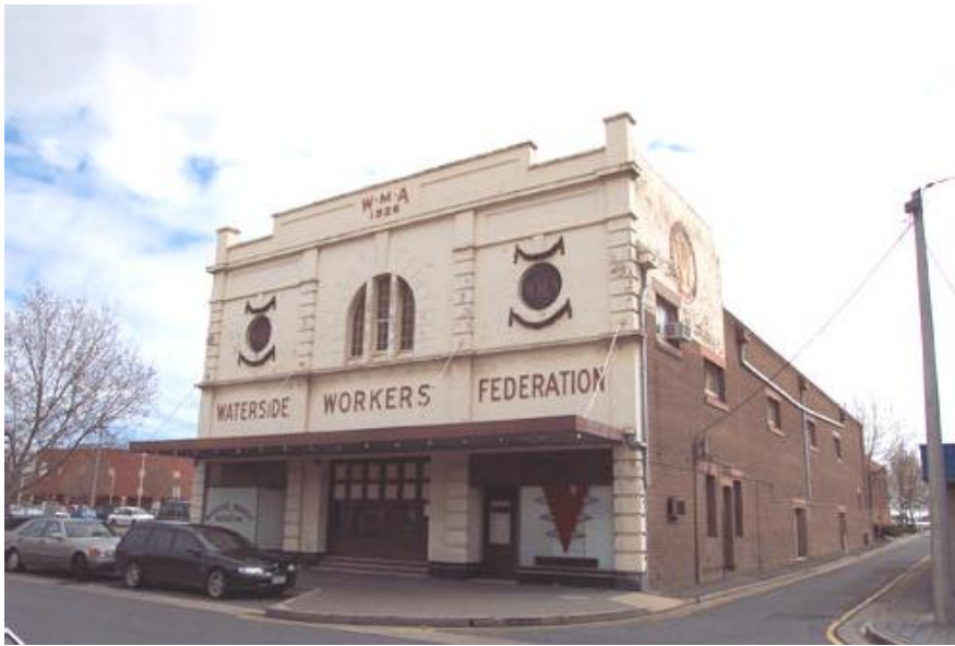
South façade, Waterside Workers Federation Hall, 2004
